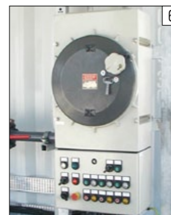
Ex-proof power panel including all switches (main switch, start/stop switch, lighting switch, emergency stop switch, etc.)
