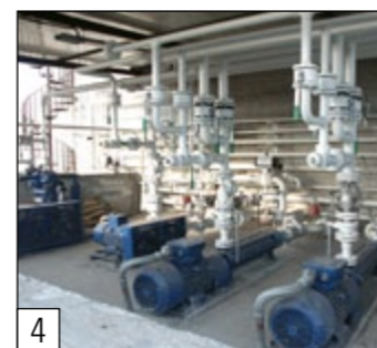
LPG pump installation
