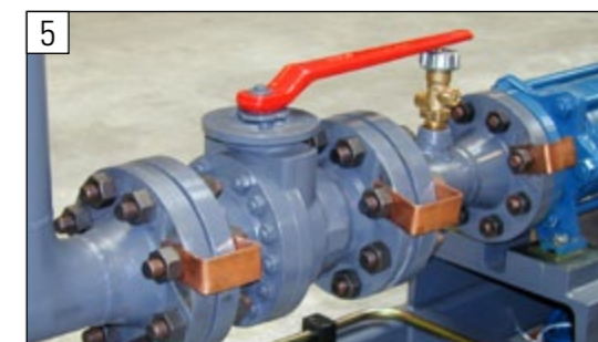
Detail of piping arrangement: shut-off valve, safety valve and earthing connections
