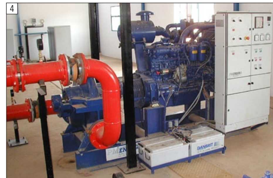
Diesel-powered fire water pump
