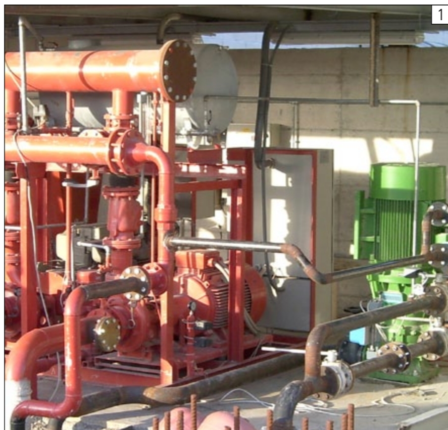
Fire water pump system
