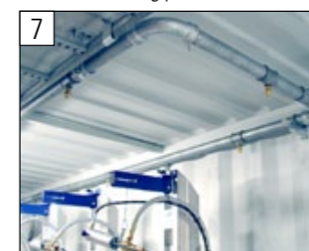
Sprinkler system integrated in container filling plant
