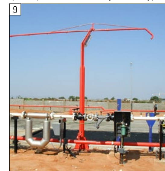
Sprinkler system at road tanker loading and unloading point
