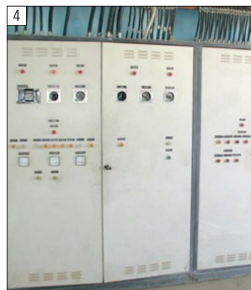
Power panel for non-hazardous area
